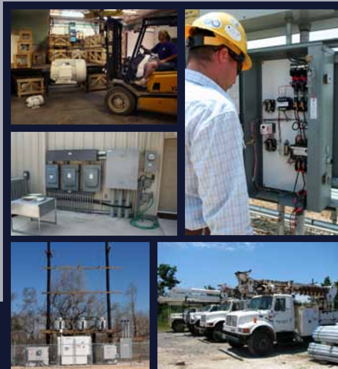
Pictured on center fold from top left: 1. REI's electrical motor stock, 2. Commercial building power distribution, 3. Troubleshooting & repairing electrical work, 4. Saltwater Disposal Power System, 5. Poleline construction equipment
